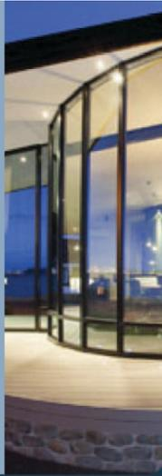
**Thermally Efficient Window Frames** - Like double glazing, thermally efficient window frames help prevent the transfer of heat energy through window frames and therefore help reduce the incidence of condensation on windows. Thermally efficient window frames should only be used with double glazing.
